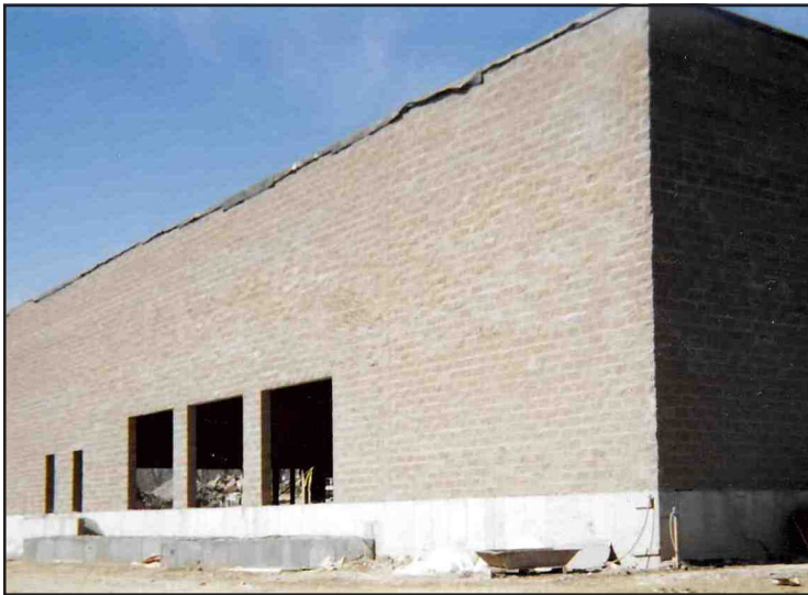
A project using split face block, Carmel, NY
