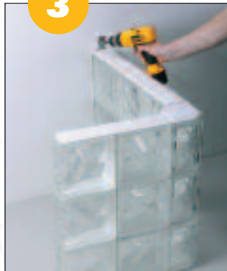
The glass blocks are secured to the wall using special wall anchors.
